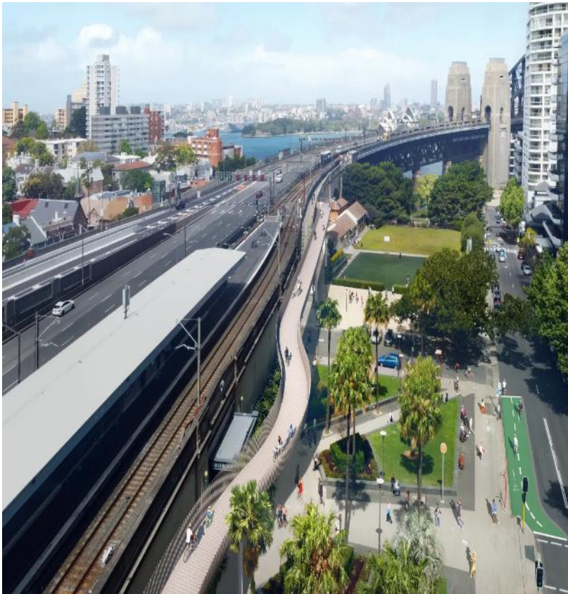
Sydney Harbour Bridge Ramp, North Sydney
