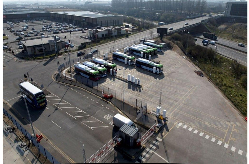
Caledonia depot, Glasgow, UK - The depot will allow over 150 buses to be charged at one time
