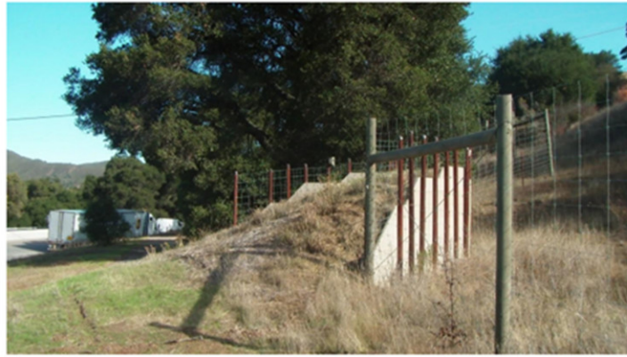
Figure 2.4.: Jumpout ramp, Highway 1010, San Luis Obispo County, California [102].
