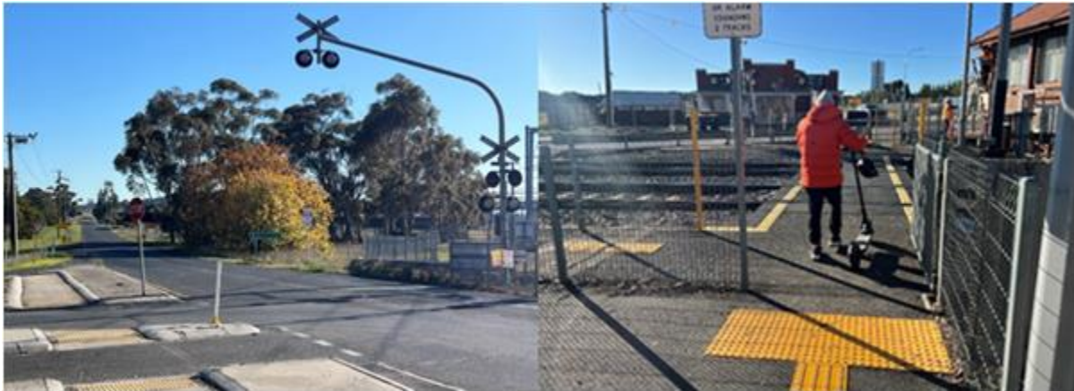
Figure 11 Diggers Rest Station Level Crossing
