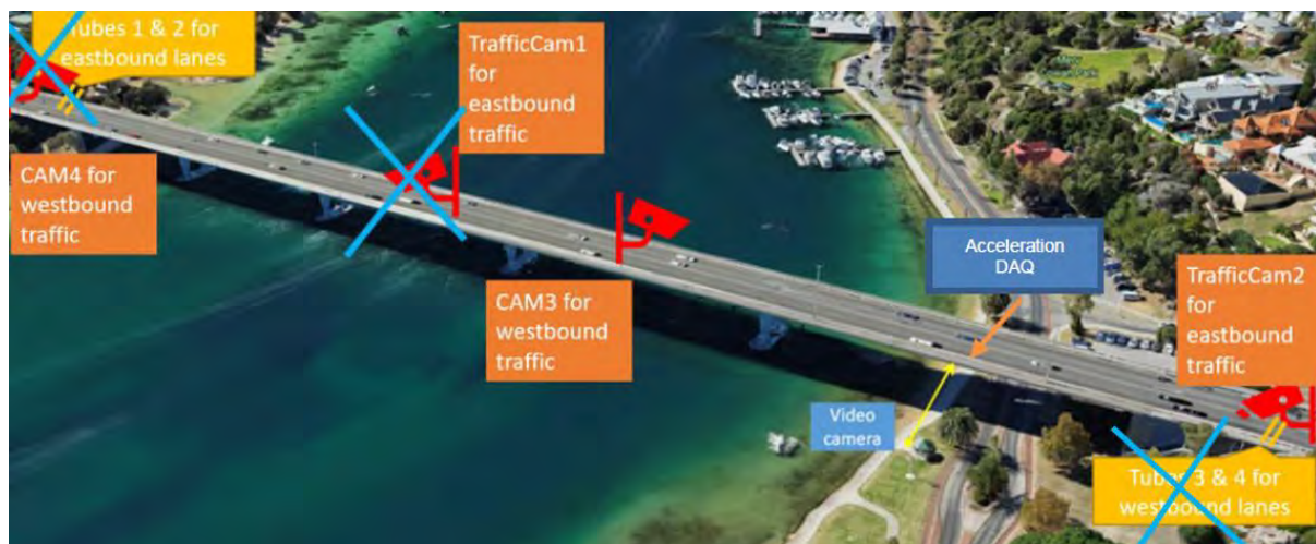
Figure 1 Traffic camera locations
