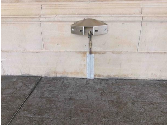
Figure 15: Restricted access to water at Central
