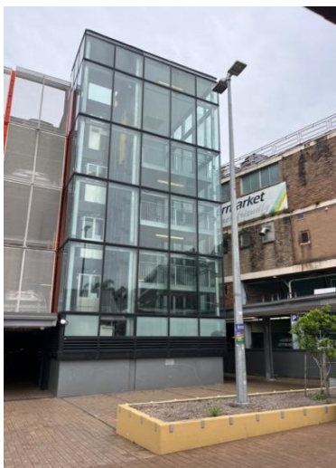
Figure 42: External carpark stairwell at Wollongong
